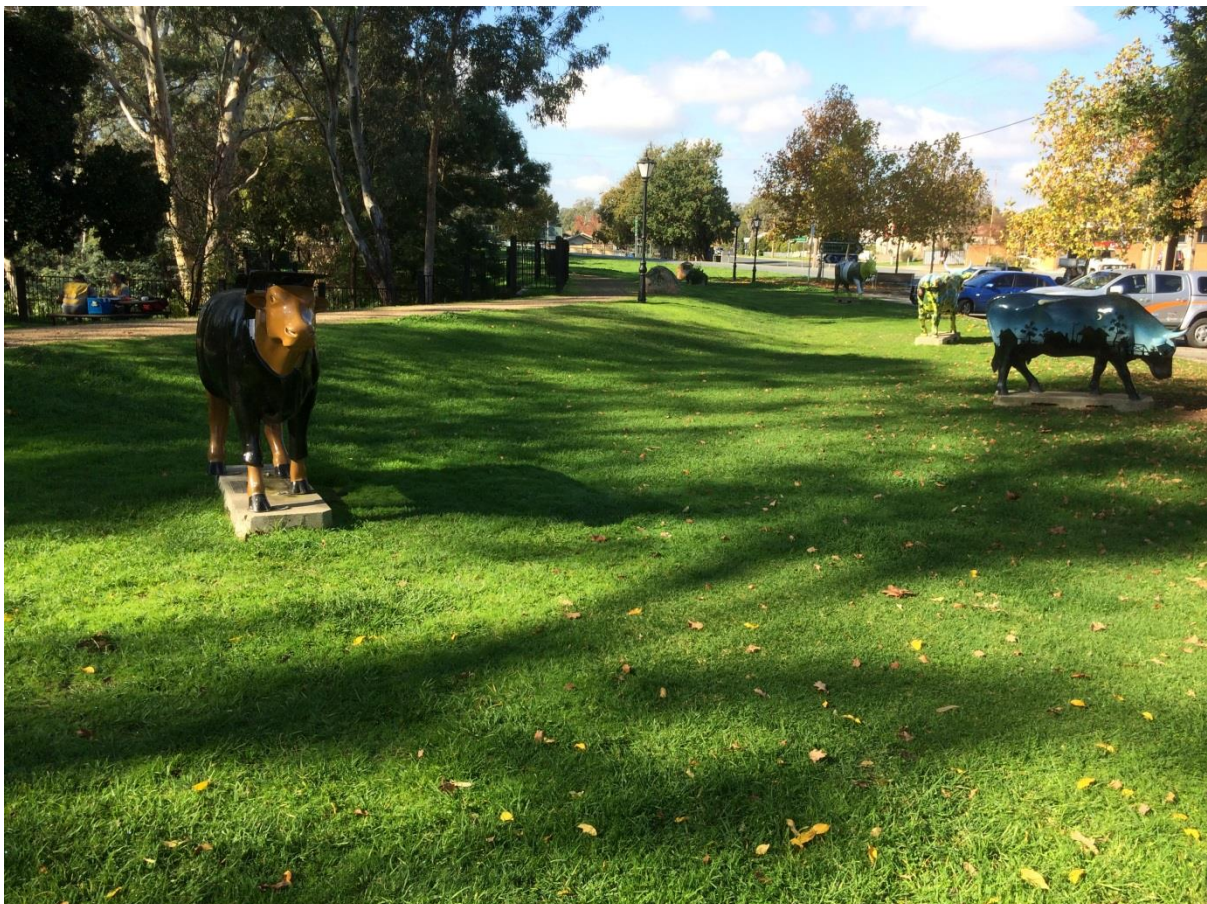
Figure 4-4 View of levee in Murchison Township looking east along Stevenson Street
